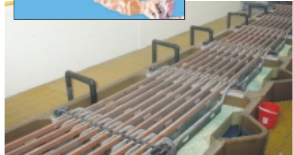
Copper-electrowinning cells in the tankhouse.
